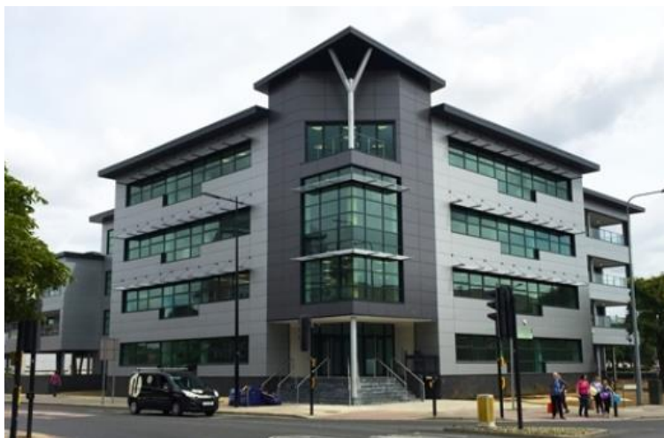
Figure 8 – Berkeley Business Centre, Connexions 159, Princes Street, Ipswich
