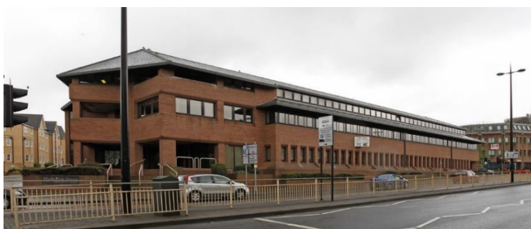
Figure 12 – Hyde Park House, 1 Crown Street, Ipswich
