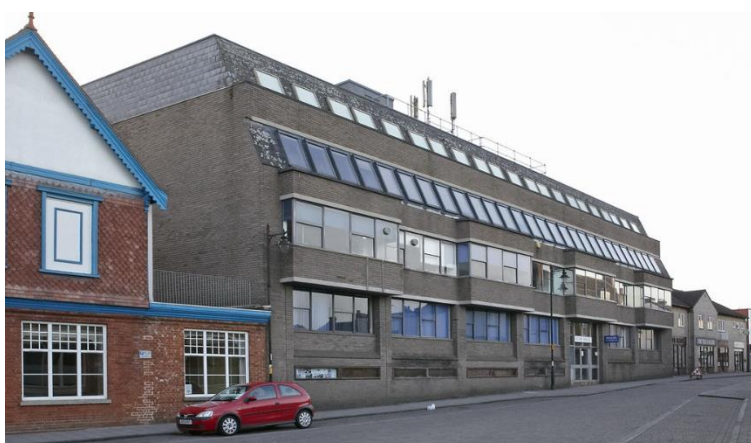
Figure 11 – Sulby House, North Street, Sudbury
